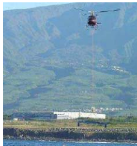
CETO 4 foundation deployment
